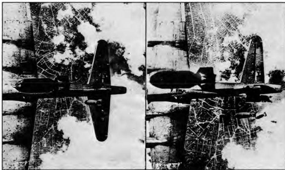
A bomb from one B-17 hits the stabilizer of the bomber below it. A deadly illustration of the importance of correct and accurate Group formation during a bombing run.
