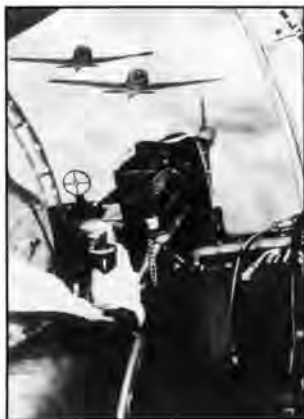
A waist gunner in a training flight in the USA. There were no bullets in his machine gun but the camera in the centre recorded where the bullets would have hit. Each crew member shot 200 feet of film from four cameras installed in the bomber.
