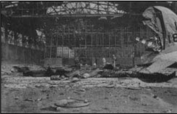
The effects of a good strafe – note the damage to this hangar – are comparable to bomb damage.
